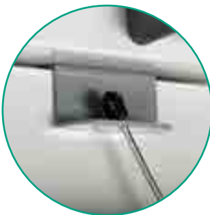
The 'hook shaped' end is trapped by the door when closed & locked
